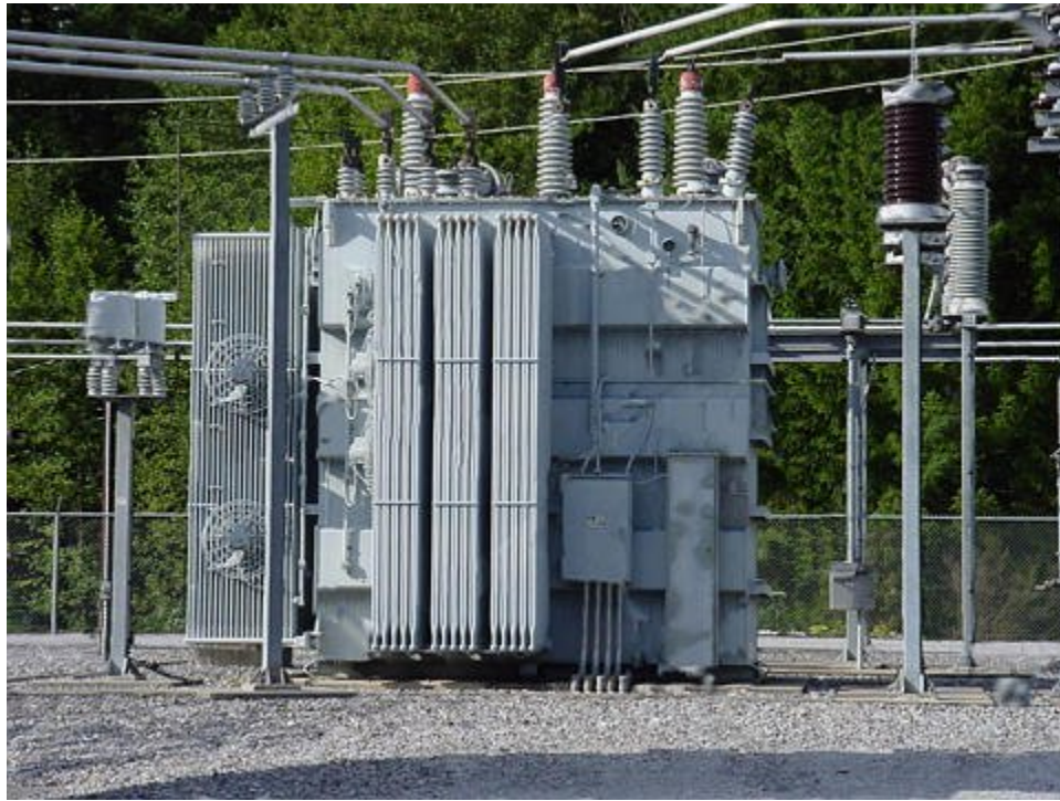
Figure 8.5 Substation transformer.
