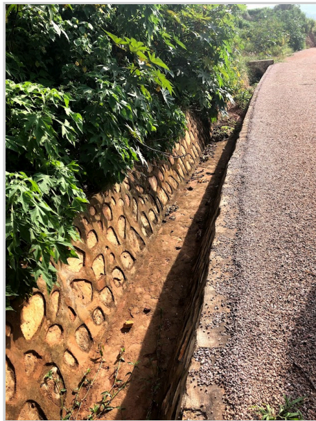
This road ditch in Uganda has complete covered the area water would run with cement and rocks so it cannot erode and undermine the road. Photo Credit: Amber Anderson.
