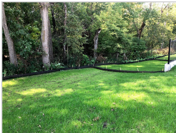
As the perennial cover of grass gets established next to the new Ames High School, these black strips are used to slow water and stop sediment moving down the hill. Photo credit: Amber Anderson.
