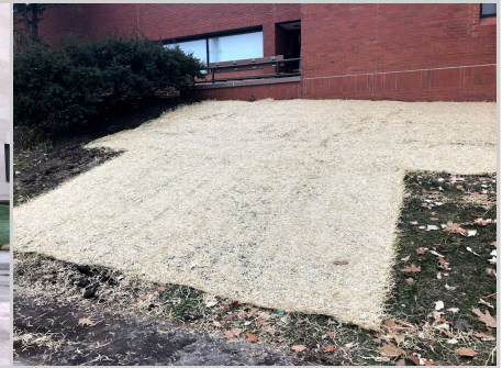
This mat is used to help protect the soil surface and keep seed in place during establishment. Photo credit Amber Anderson
